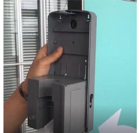
Hook sanitizer dispenser onto the screws of the connector
